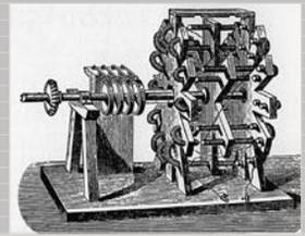
First 'working' electric motor.
