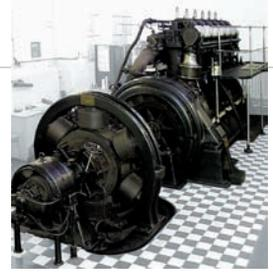
In 1918, a three-meter high, decommissioned submarine motor was procured as an emergency generator. It still stands in one of the factory buildings.
